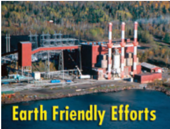
Taconite Harbor generating station
