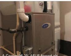
A Carrier 96.2% AFUE forced air gas furnace with an ECM, recently installed in a Duluth-area home.
