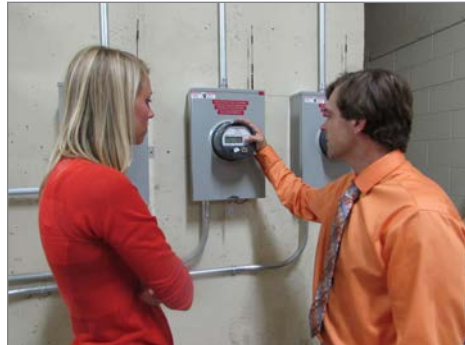
Katie Gascoigne and Paul Helstrom check output of PV panels on the Government Services Center
